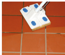
Apply solution to the surface with a mop or sponge. Under floor heating must be off.
