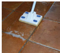
Apply solution to the surface with a mop or sponge Under floor heating must be off.
