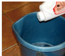
Dilute Grout Stain Remover 1:3 with water.
